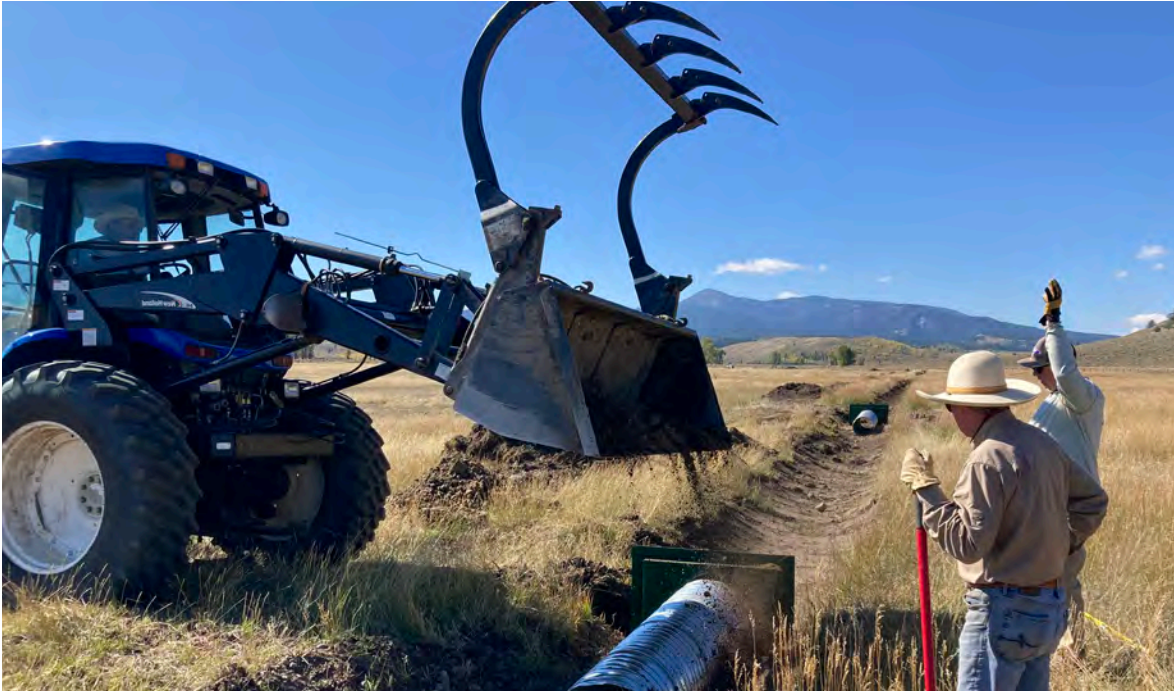
Placing fill at the new headwall at Elk Ranch
