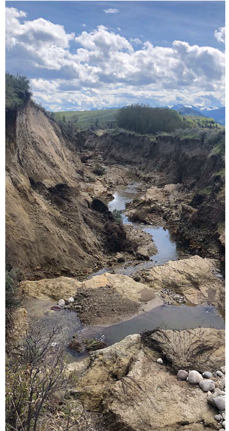
A blownout South Park supply ditch in the National Elk Refuge
