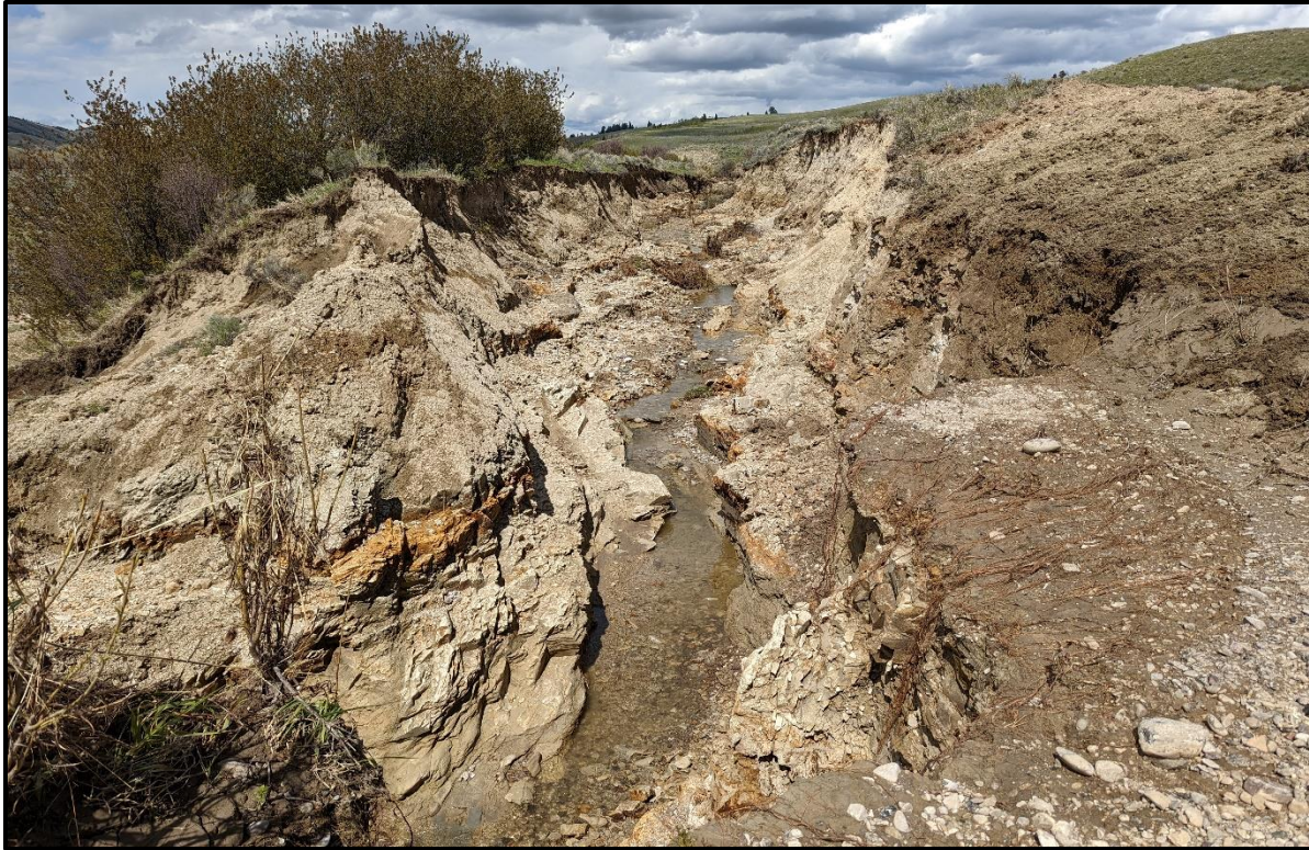
Figure 8: Ditch breach looking upstream from the original ditch location. Breach in center left.
