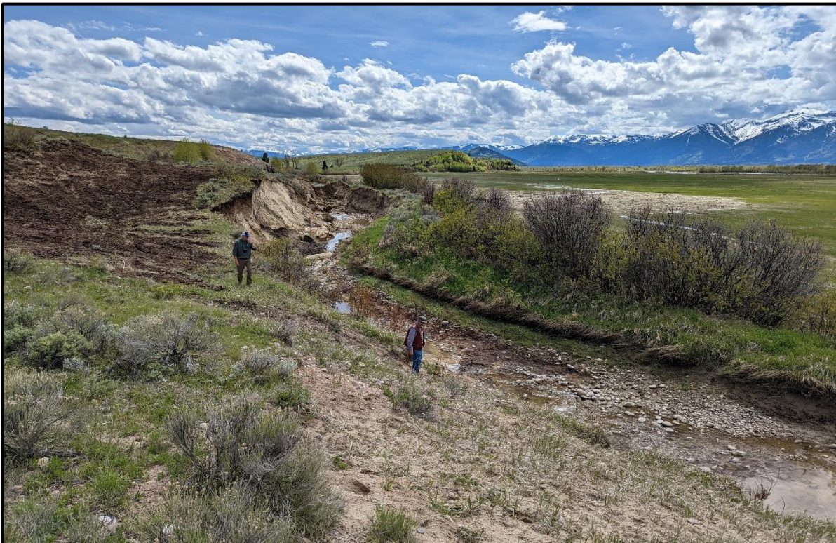
Figure 7: Ditch failure. Photo taken from left bank, looking downstream. Debris fan visible in top-right.
