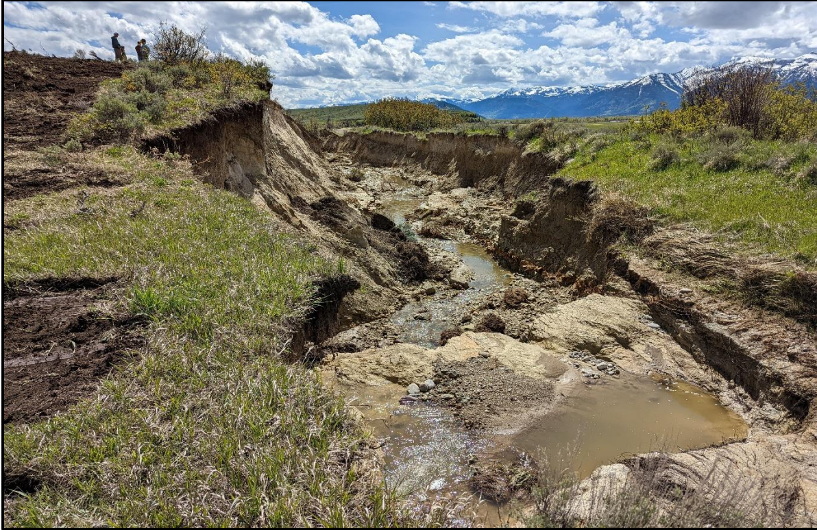
Figure 6: Failure of South Supply Ditch, looking downstream. TCD Staff visible in top-left.
