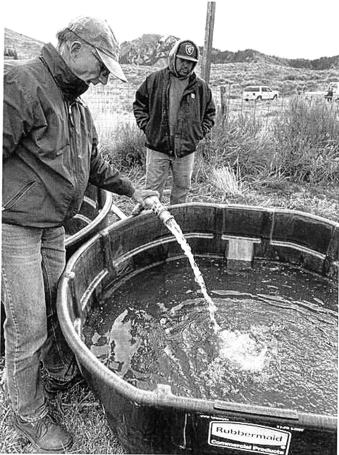
Photo 3. Picture Taken at Beginning of Pump Test. Flow Measured at 10 gpm with Bucket and Stopwatch.
