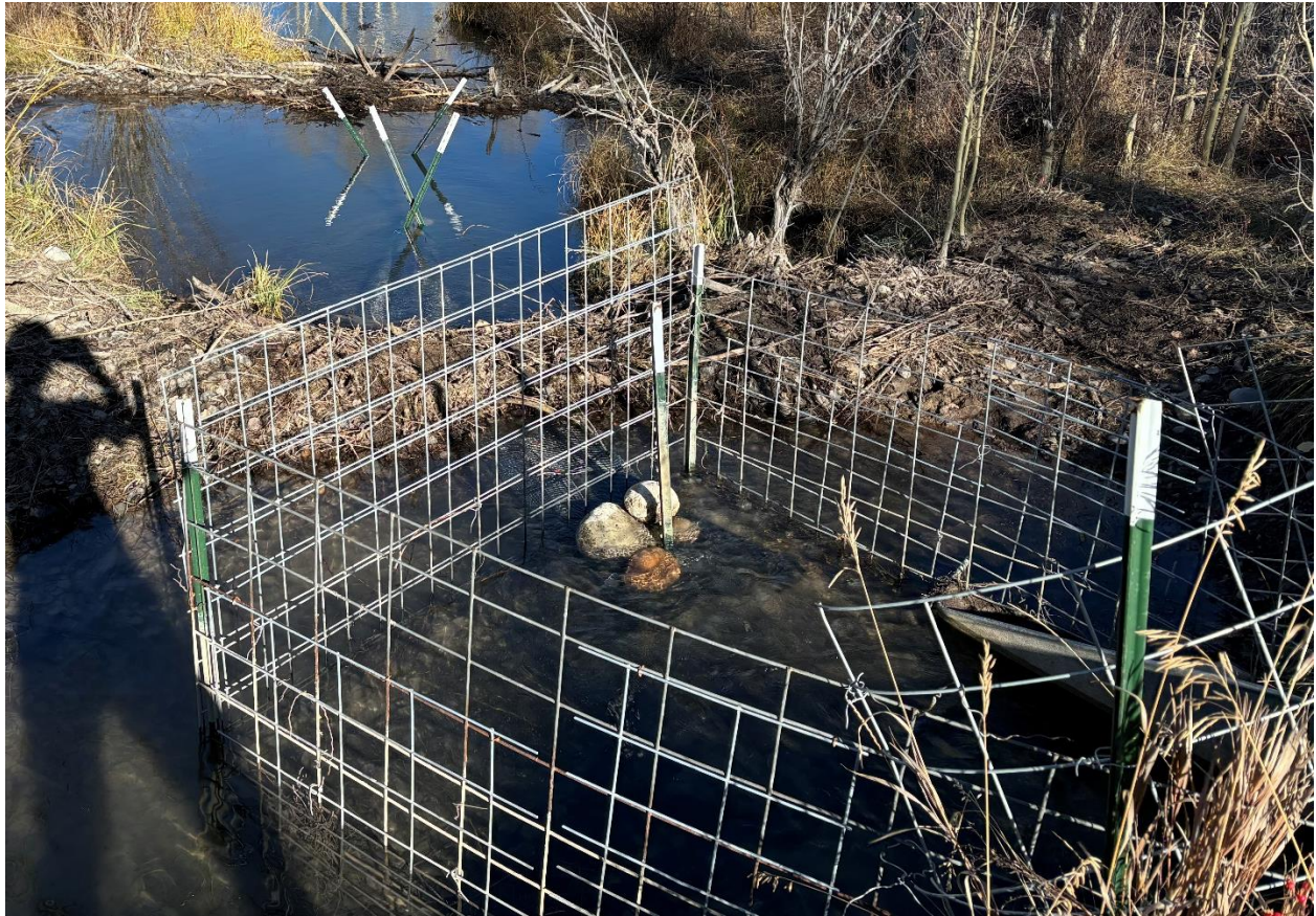
Culvert Fencing on Alkali Creek. Some pond leveling tubes are installed on the downstream side.
