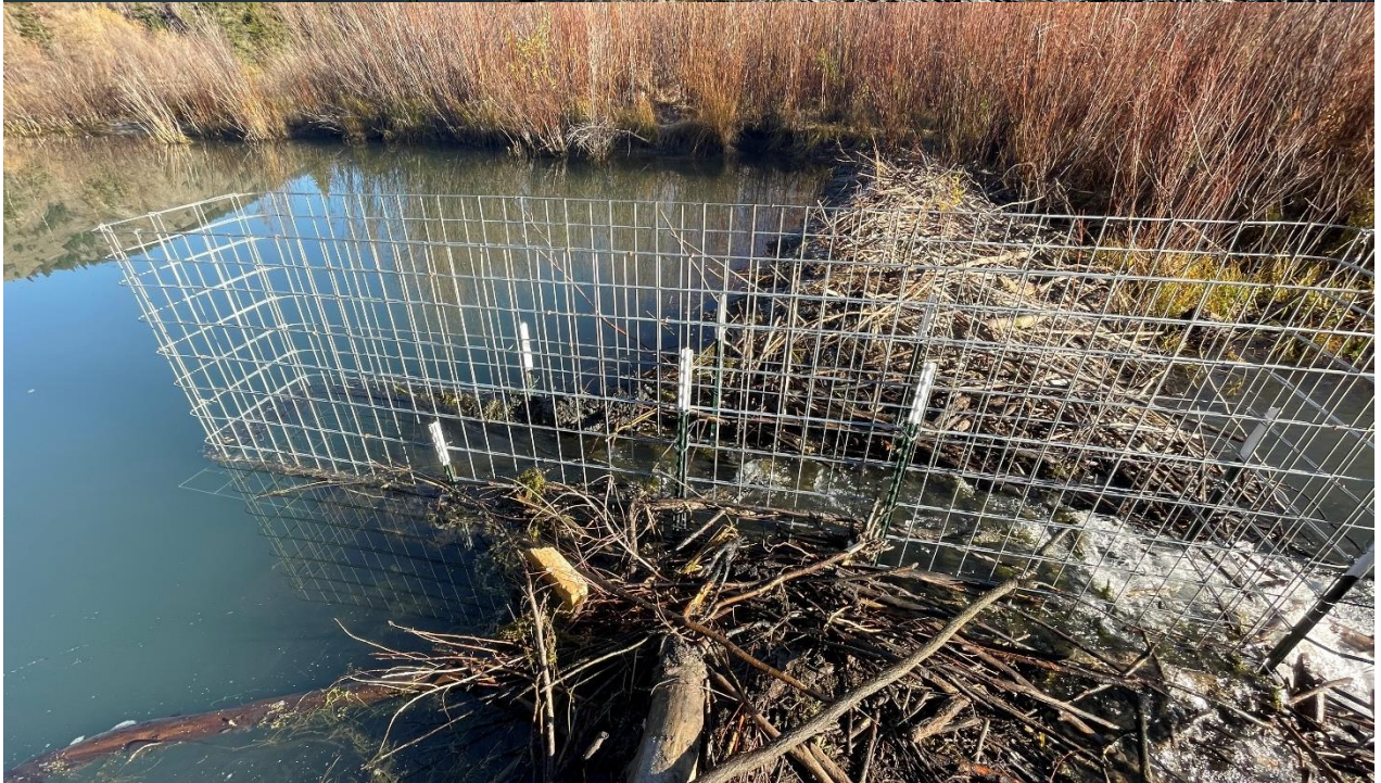
Dam Notch Exclosure Fence, another kind of pond leveler, on Dog Creek, excludes beavers from the break in their dam allowing for a lower pond level.
