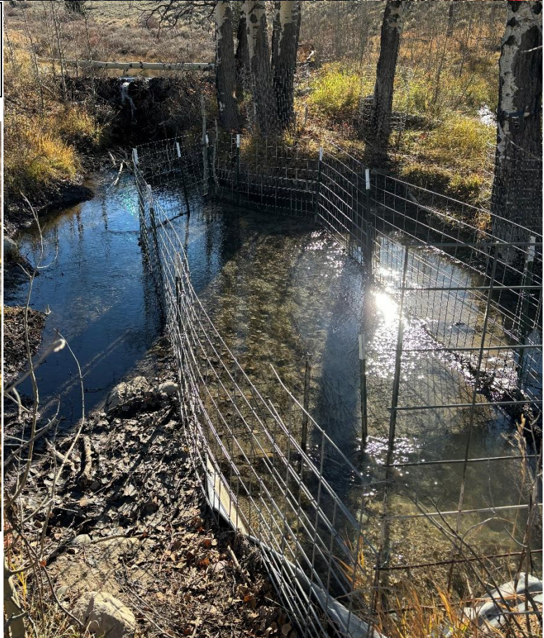
Culvert Fencing on Alkali Creek. Some pond leveling tubes are installed on the downstream side.
